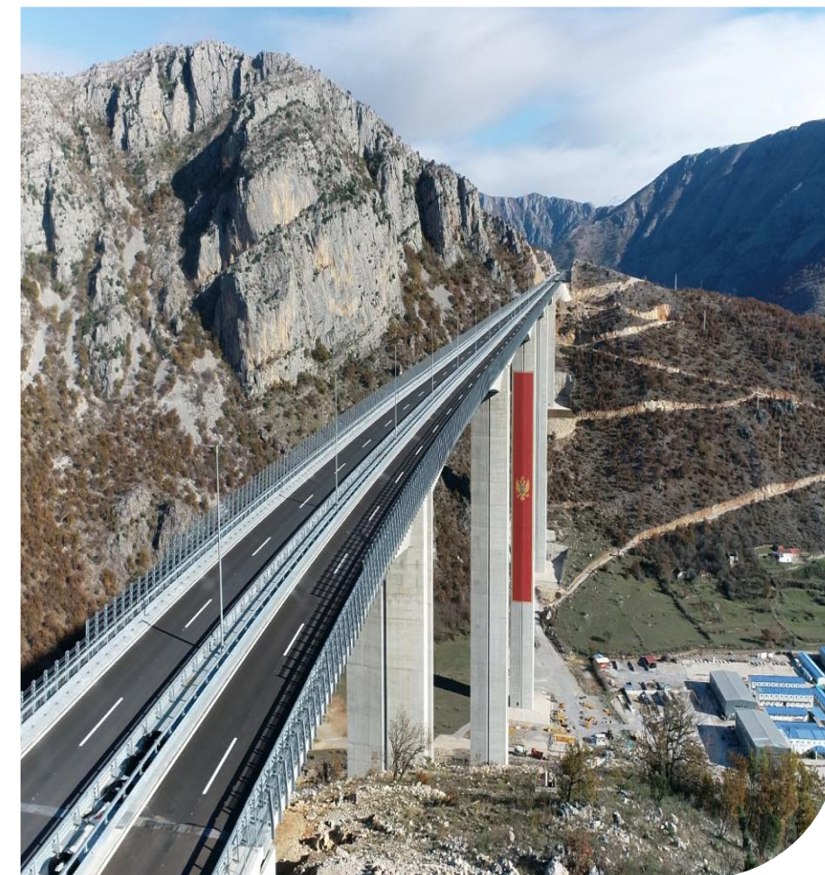
Moračica Bridge, Podgorica, Montenegro
